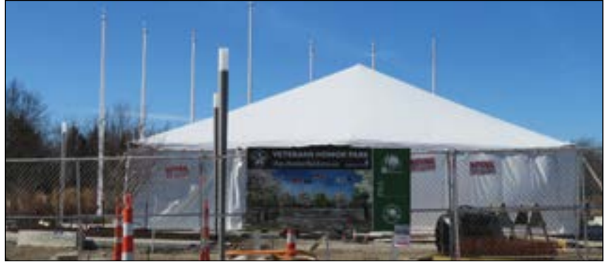
The flagpoles and star monument currently under construction at the park.
